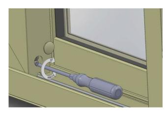
Verify that the installed door is flat, plumb, level and square. Verify that the door is shimmed and fastened properly as stated in these instructions.
